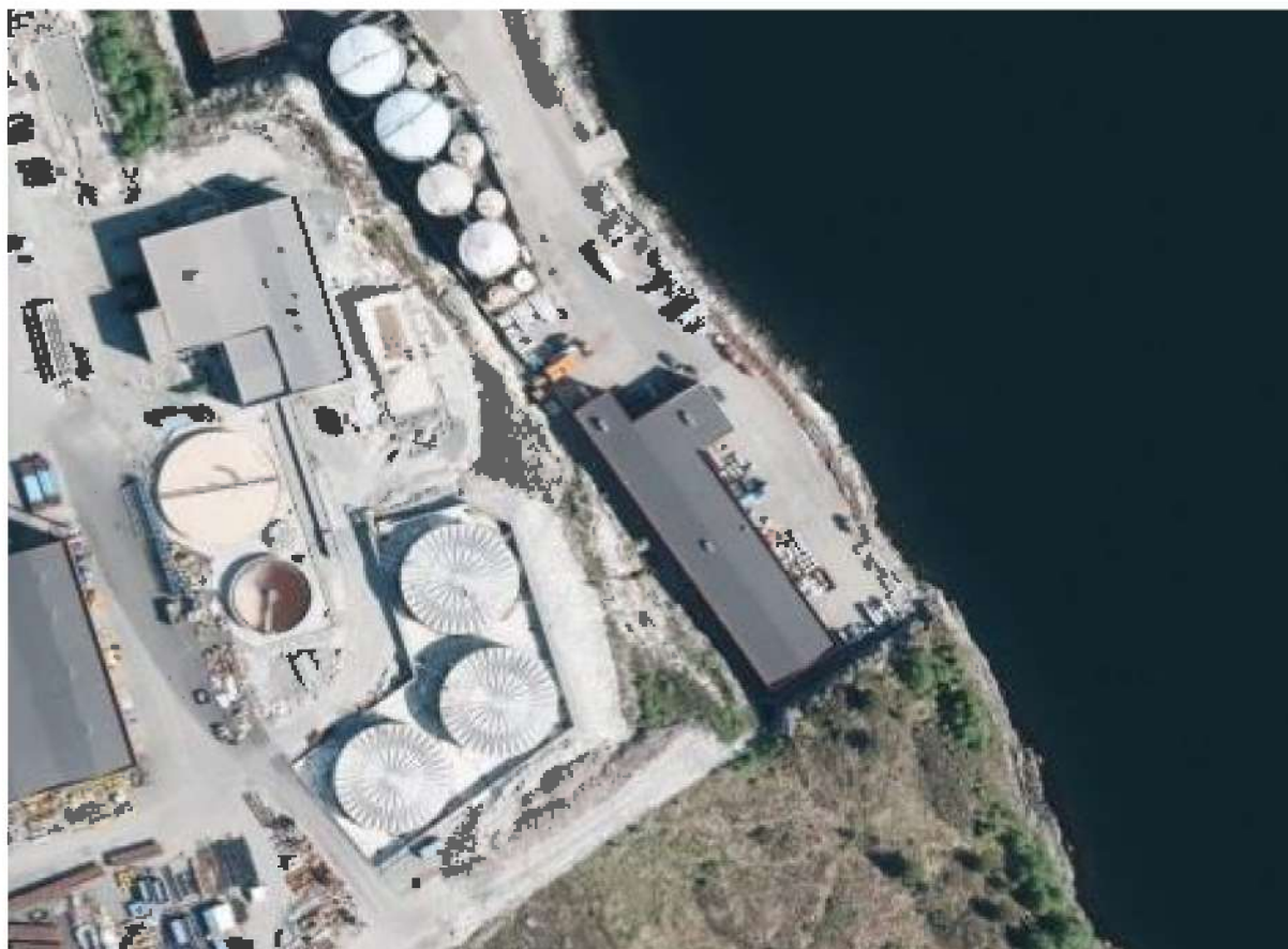
Bilde 1 Oversiktsbilde over Mongstad Treatment Plant
