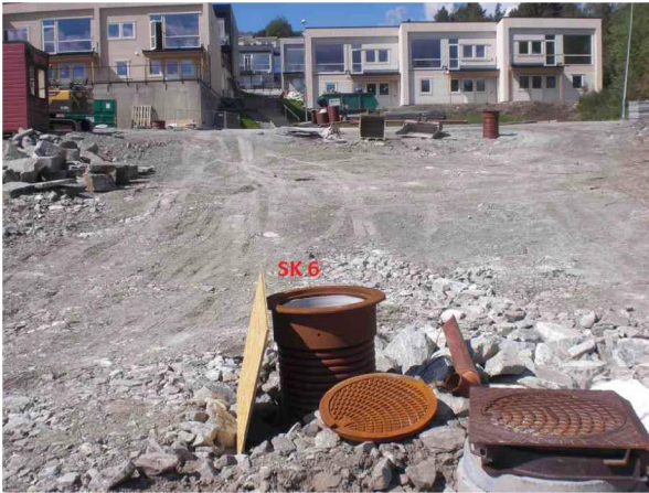
SK6SK728052108291B.jpg, 00:00:00, 0.00m Start inspeksjon / i SK6
