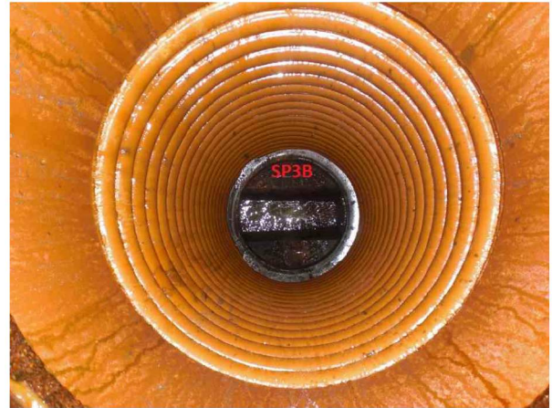
L26.11.2021 102917_SP3B_SP3A_261121_104141_9.jpg, 00:00:00, 0.00m Start inspeksjon / i SP3B
