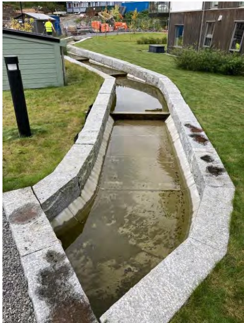
Figur 6, åpen renne for overvasshandtering.
