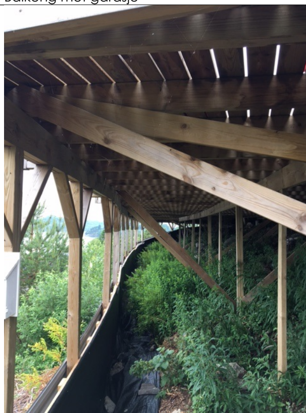
Terreng under terrasse
