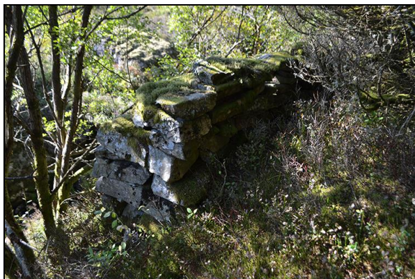
Fig. 35: Steingard N 14 sett mot V.
